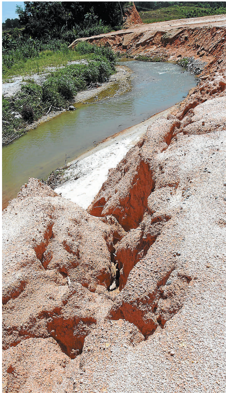
Slip sliding away: The bank of this stream is on the verge of collapse, raising the risk of flooding and mudslide.
