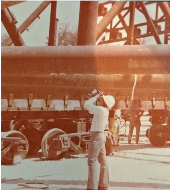
Risky under the platform.
